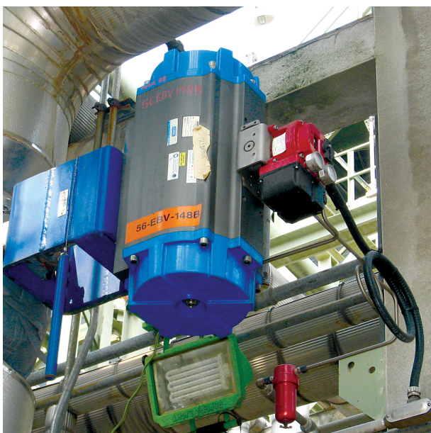
Figure 2. Emergency shutdown digital valve positioner.
